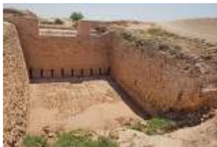
Ancient Water Treatment Facility
